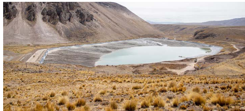
▲ Caylloma Mine tailings storage facility
