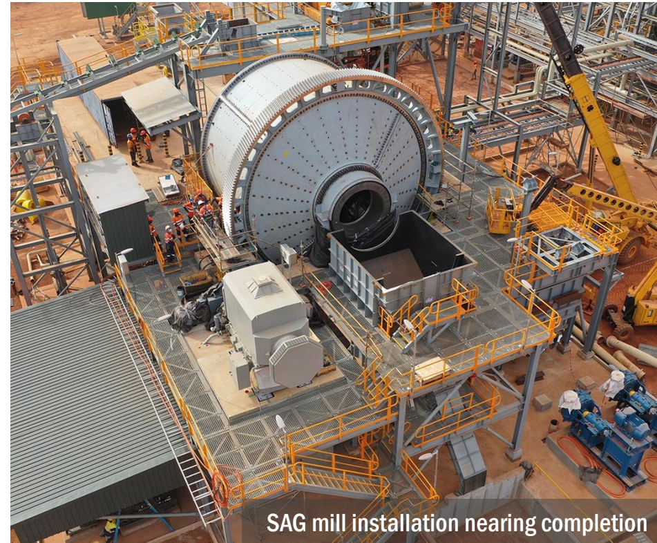
ROM bin and crushing circuit installed
