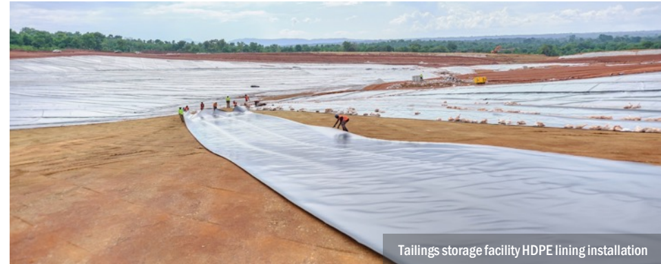
Tailings storage facility HDPE lining installation
