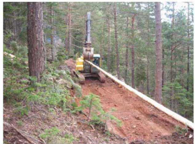
Drill road construction
